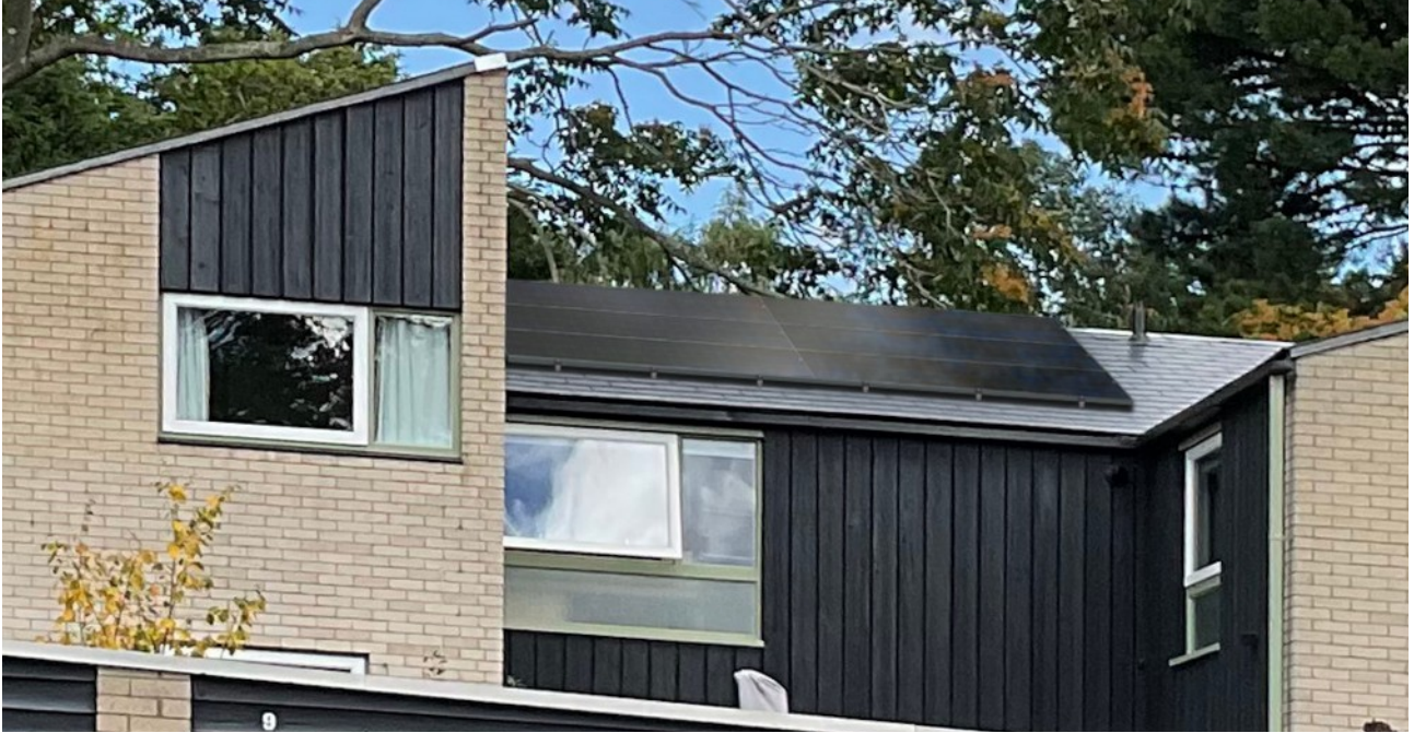
Figure 2: Detail showing one house with panels
