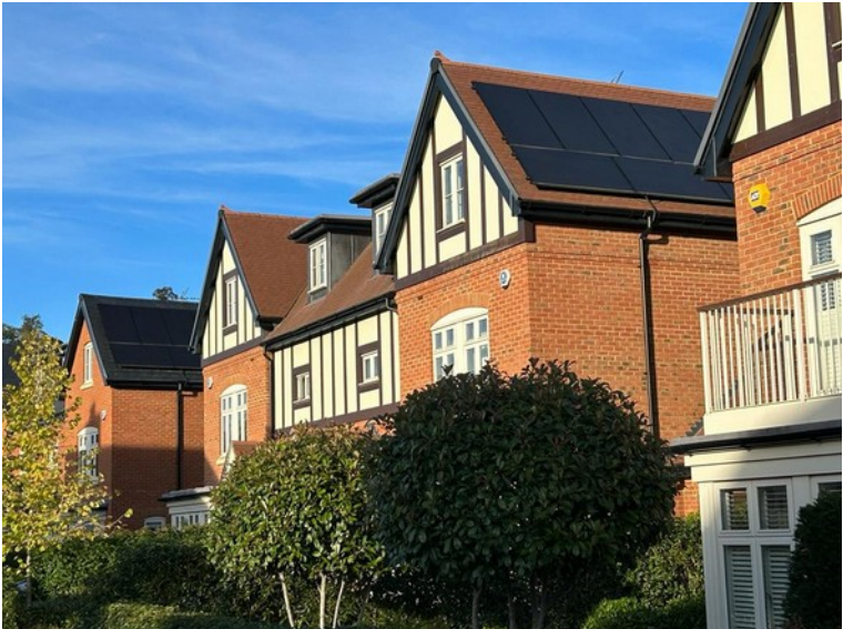
Figure 4: Two Mill Lane houses with black panels: note the one on the left which has dark slates
