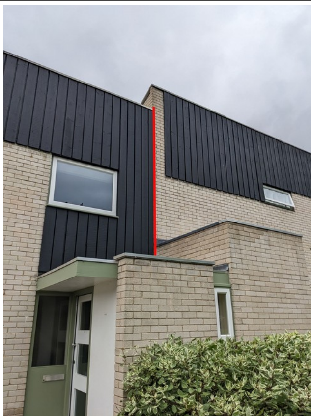
This route is most useful for the house on the right as it goes straight down to the utility room
