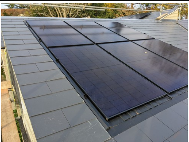
Panels mounted in-roof
